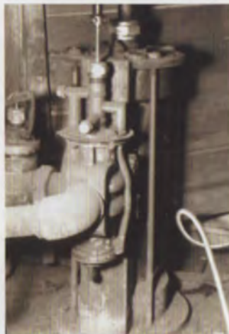
The water motor installed in 1880 to blow the S. R. Warren Organ in St. Michael's Cathedral. It operated on fifty pounds of water pressure. The large diameter pipe is a drain pipe. The large rod at the top is driven by a double-acting piston and is connected to a rocking lever and two 'feeder bellows'.
